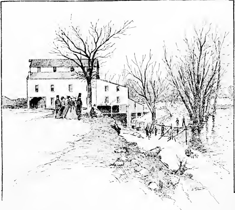
THE RUDISILL MILL.
